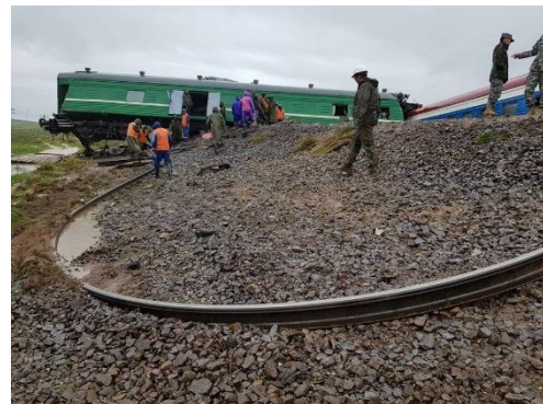
Figure 12-3 Flooding in Sainshand and damage to the railway due to flooding near Airag soum
